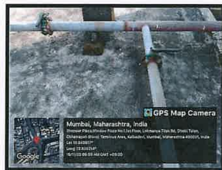
Waste Water In Seepage Tank
